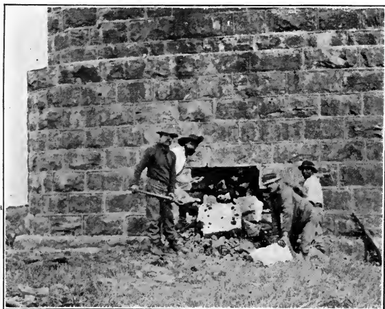
Colonel Ricardi of the Dynamite Brigade superintending the covering up of the dynamite charge before firing.
